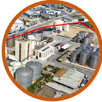
Rainwater recovery system
