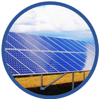
Installation Of solar panels
