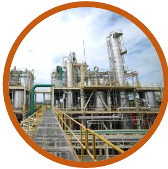
Naturally created biogas
